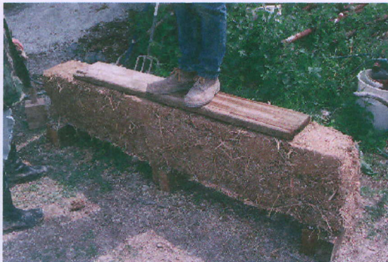
Figure 3. Building a Cob Wall
