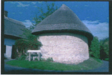
Figure 1. Cob Walling Construction in England
