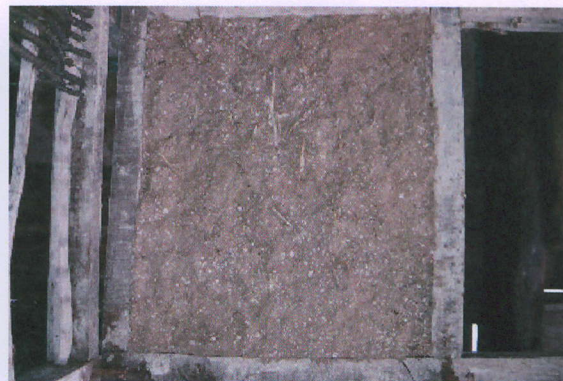
Figure 7. Wattle and Daub Wall Construction
