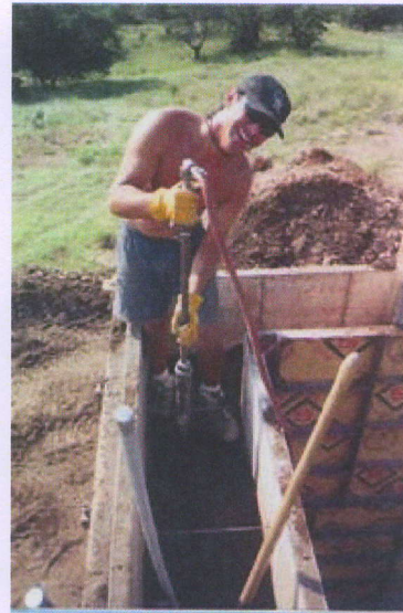
Figure 2. Rammed Earth Construction in Arizona (Photo courtesy of Rammed Earth Development Inc. at http://www.rammedearth.com/ )
