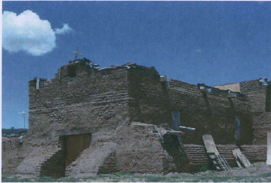
Figure 4. Adobe Church in New Mexico
