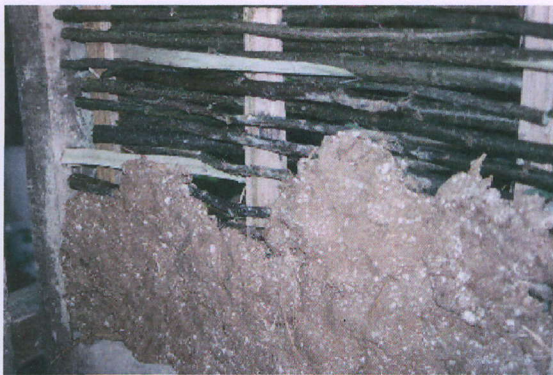
Figure 6. Wattle and Daub Wall Construction
