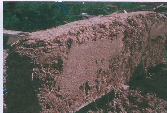
Figure 2. Rammed Earth Construction in Arizona (Photo courtesy of Rammed Earth Development Inc. at http://www.rammedearth.com/ )
